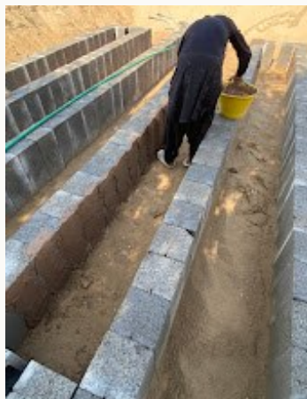
Manual construction and sealing work.
