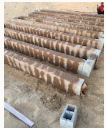
Rows of the first concrete-block prototype.
