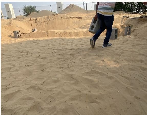
Prepared field area and watering lines.
